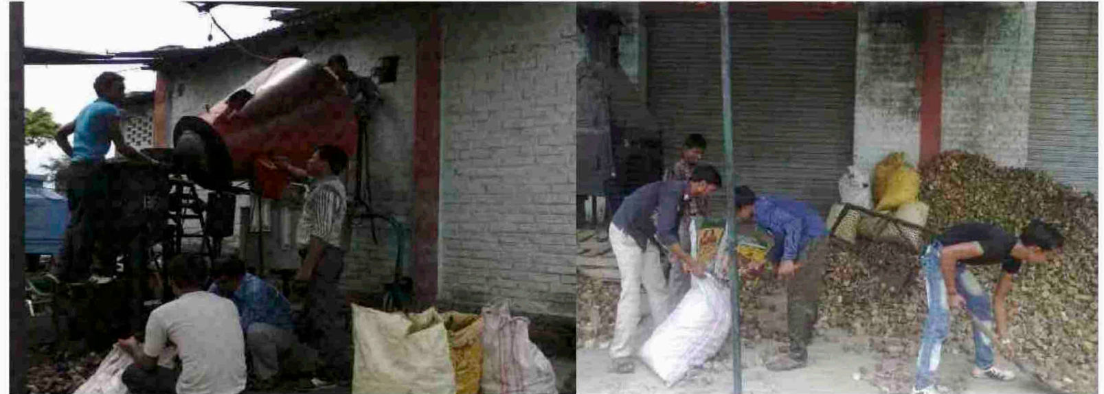
On job training at site
